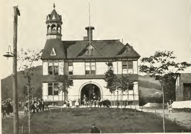
OLD SCHOOLHOUSE IN DISTRICT 17. SOUTH ROYALTON GRADED SCHOOL BUILDING.
